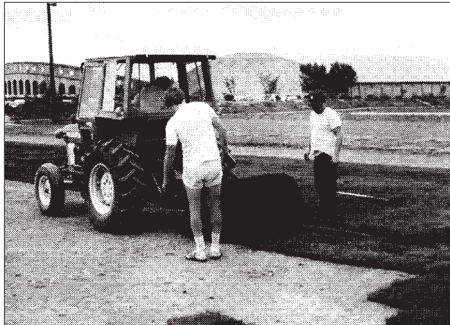
▲ A sod installation at Cornell University.
